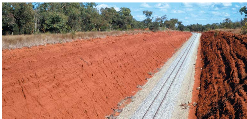
Deeply weathered Red Kandosol, Pentland railway cutting, north-central Queensland
