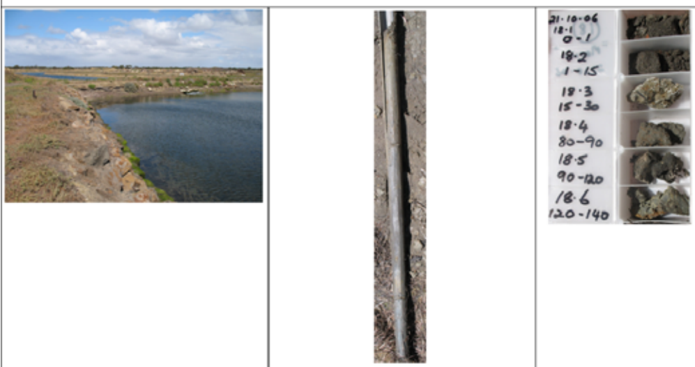
Embankment, unauthorised marina, Drysdale COR 18: Natric Sulfidic Intertidal Hydrosol
