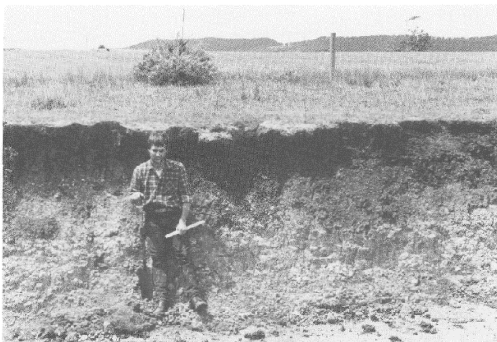
Streambank erosion in the Apsley River Flats (394122} Land System
